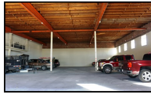
Parking Structure at The Mercantile
